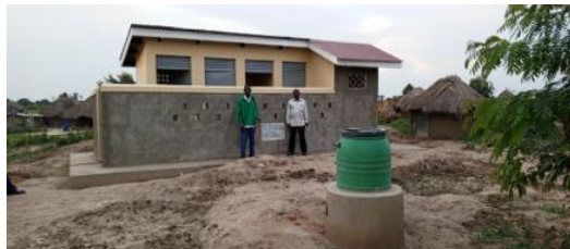
Figure 3.1: The LC1 chairman and his Vice posing in front of newly constructed pit Latrine in Kabolwa trading centre.
